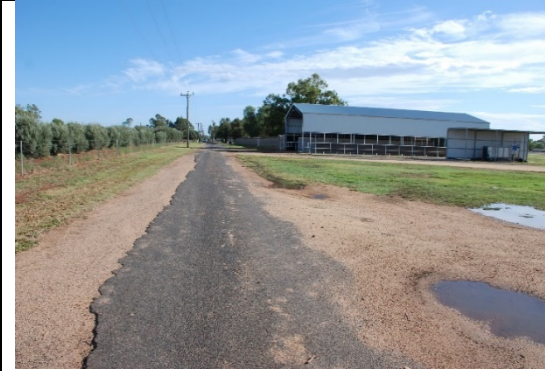
Plate 24: Internal driveway looking north on western side of site
